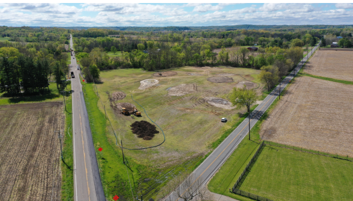
Henshaw Wetland Under Construction
